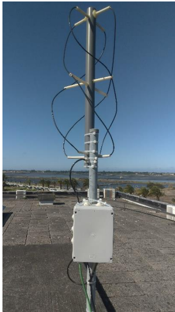
Fig. 1 NOAA satellites receiver setup
